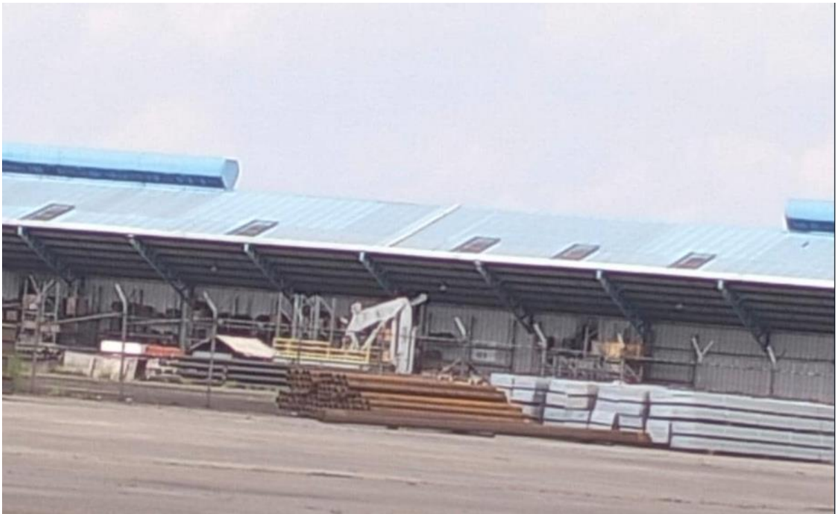
Delivered Structural Steel Pipes
